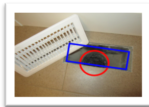
Figure 5.a. Air Duct Tubing ( Red ) and Air Vent Register Interface ( Blue )
